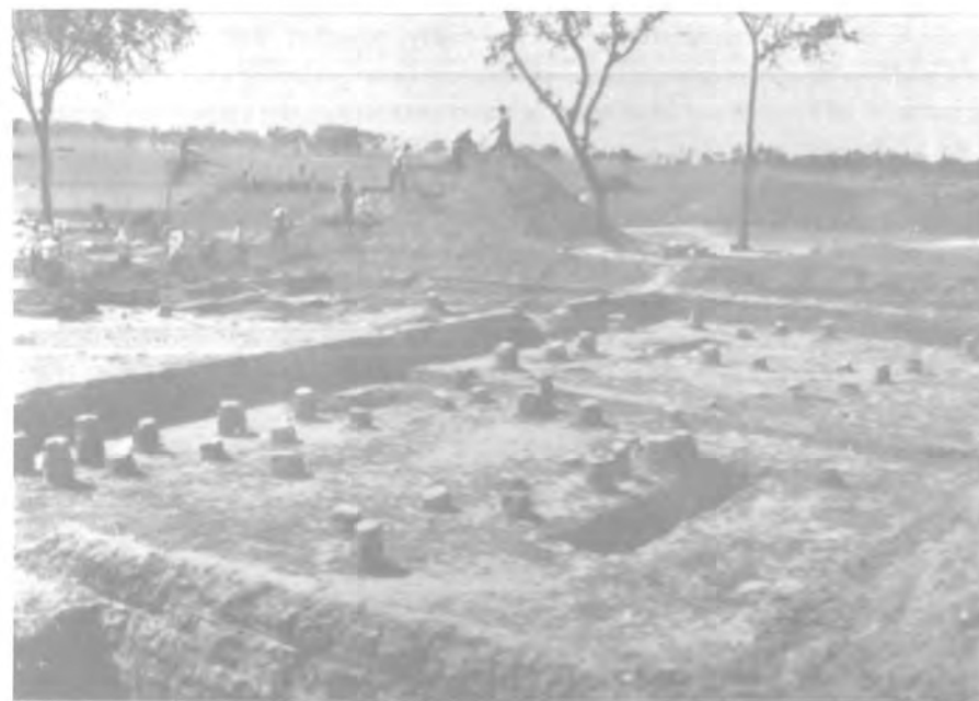
278. The stamped-earth floor with stone post bases of a Shang house at Hsiao-t'un, An-yang. (From Shih Chang-ju, Yin-hsü chien-chu yi-ts'un , 1959, pl. 9.)
