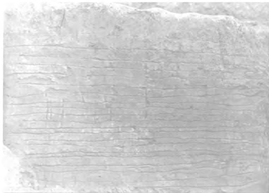
277. Side view of stamped-earth layers of a Shang house floor at Hsiao-t'un, An-yang. (After Shih Chang-ju, Yin-hsü chien-chu yi-ts'un , 1959, pl. 11.)
